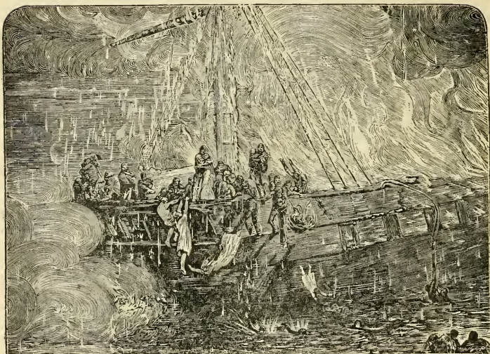
The Scene, two hours after the Fire was discovered.
